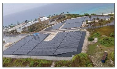
The Energy Conservation Measure shown above includes 2,380 kWdc of solar Photovoltaic electricity generation, 2 MW/3 MWh lithium-ion battery Energy Storage System and microgrid control system on the island of Meck, in the Marshall Islands. This reduces the island's dependence on diesel fuel electricity generation by an average of 55 percent throughout the ESPC performance period and provides energy resilience to critical missions located in the region.
